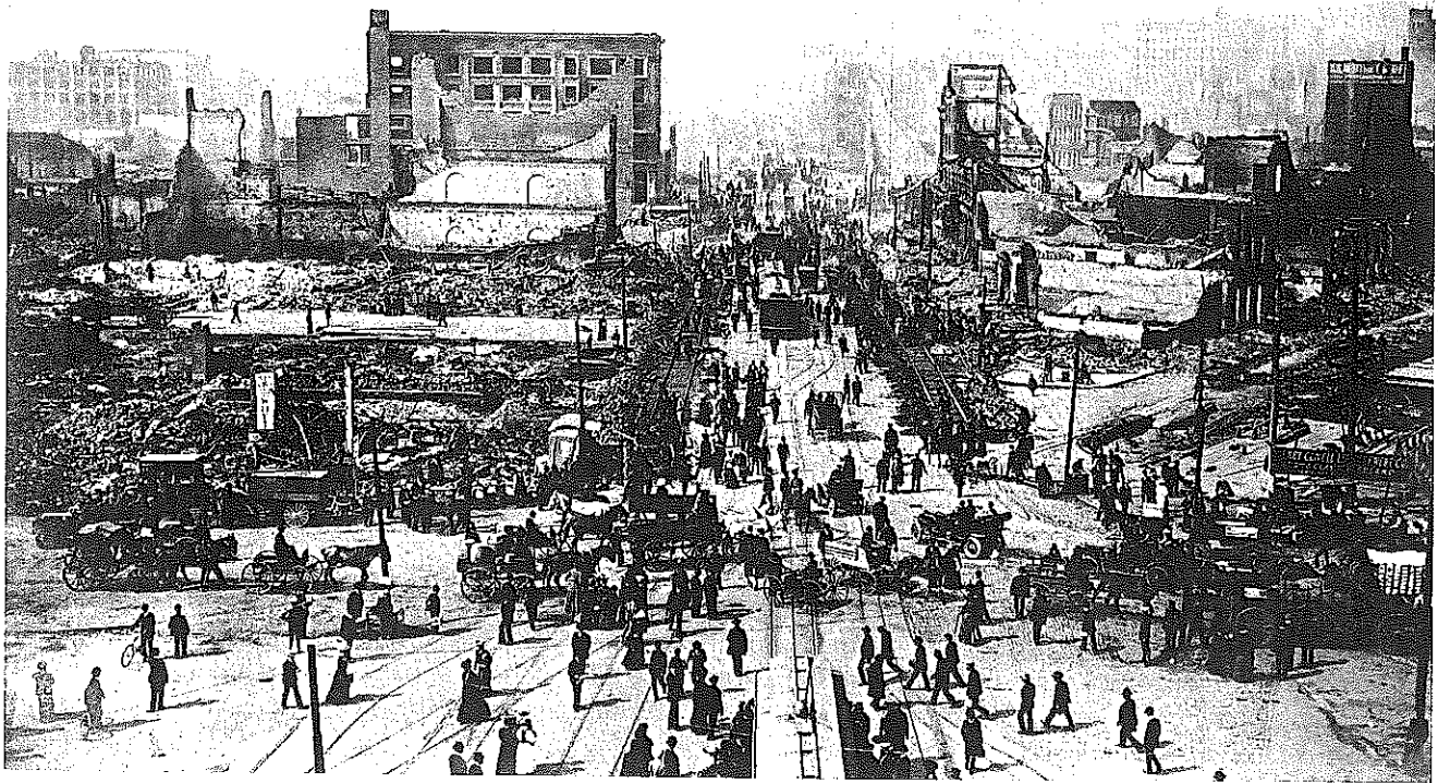
Figure 3.20 Destruction from the San Francisco earthquake and fire. The first shock struck San Francisco early on the morning of April 18, 1906, damaging the city’s water system. Fire broke out and raged for three days. It was finally stopped by dynamiting buildings in its path. When it was over, some 700 people were dead or missing, and 25,000 buildings had been destroyed. Locally, the event is usually referred to as the Great Fire of 1906, suggesting a denial of the natural hazard in favor of assigning blame to correctable human error. Post-destruction reconstruction began at once. Rebuilding following earthquake damage is the general rule.
